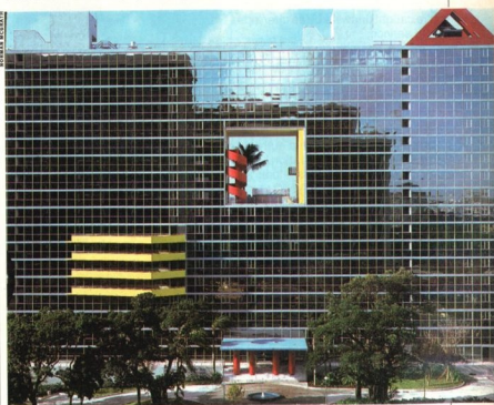
Atlantis condominium in Miami with "sky court": exuberance that is still functional
